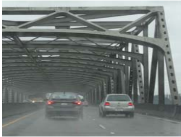
Before photo of bridge design. Image posted to Flickr by ossguy.
